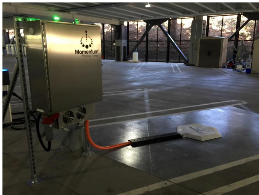
Fig. 15. Clustering high-power WPT (50-kW GA pad shown).
