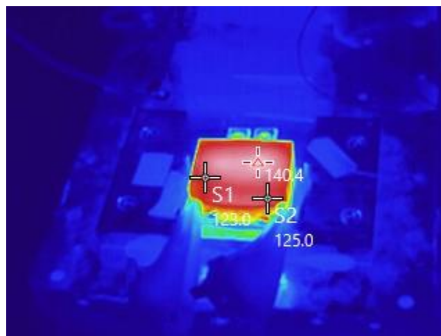
Figure. The hot spot temperature is a critical factor in determining component failure rate and MTBF of planar transformers. In this example, we measured a surface temperature of 140.4°C on the transformer.
