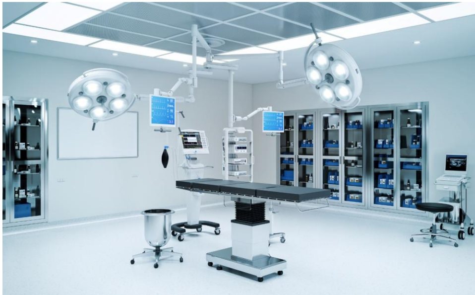
Fig. 1. In medical environments such as operating rooms, power supply requirements are complex both in terms of electrical specifications for voltages and currents, but also with regard to the approvals needed to ensure the safety of equipment operators and patients.
